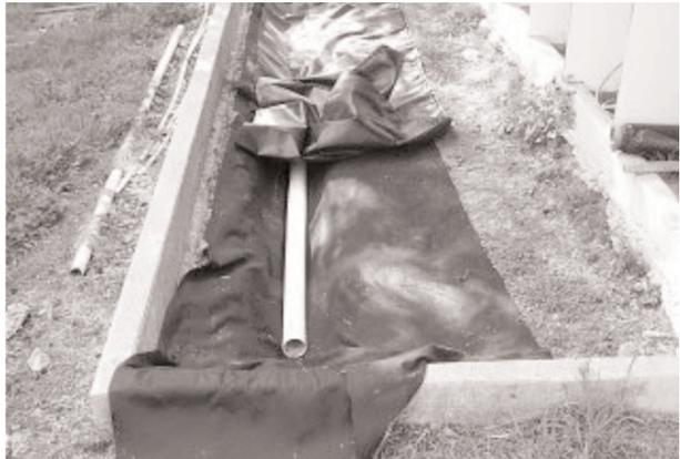
Picture showing underground drain line for outside flights. It is set in and covered with filter fabric. The fabric is used to keep the finer pieces of gravel from getting into the pipe.
