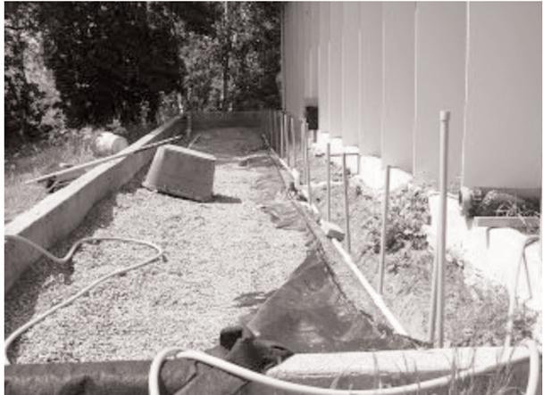
Picture showing the water main line with the services coming up at each flight. This area gets covered with gravel to within 2 of the foundations.
