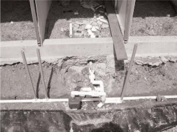
Picture showing the incoming water, a master shut off valve by the foundation and the battery operated timer for the mister system, which is stubbed up on the right side of the picture.
